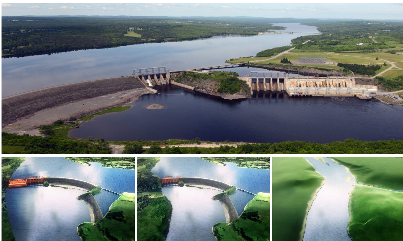
Figure 11: The Mactaquac Hydroelectric Generating Station Dam (actual current view- top) and the options considered for its renewal/removal: Repowering (construction of the new powerhouse and other components – bottom left); Maintaining the dam as a water control structure without power generation – bottom middle, and Removing the dam to ensure a free-flowing river - bottom right Credit and Source: New Brunswick Power 2013; https://www.nbpower.com/en/about-us/projects/mactaquac-project/resources/
